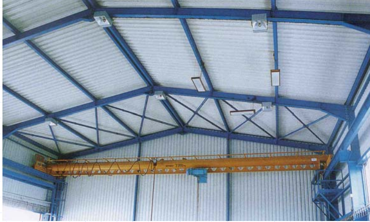
Roof bracing of a single-storey industrial building
