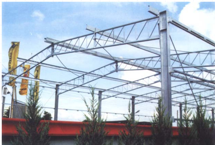
Trusses of a single-storey industrial building
