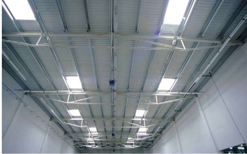
Trusses of a single-storey industrial building
