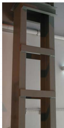
Battened column composed from two channels
