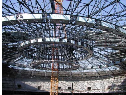
Trusses of Sazka Arena (now O2 Arena) in Praha Vysočany
