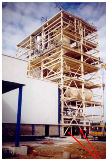
Industrial building - technological platform
